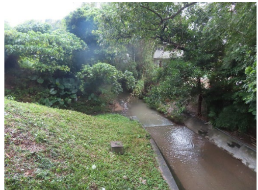
Proposed Drainage Works Area of Ha Che (CH.A 653.949 ~ CH.A 905.63) Date taken: 22 nd November 2023
